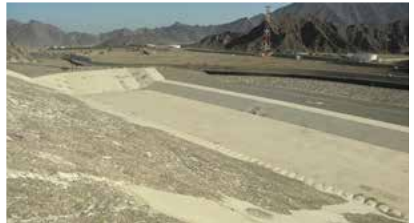
Spillway natural rock-chute and reinforced concrete stilling basin at Wadi Wurraya Dam
